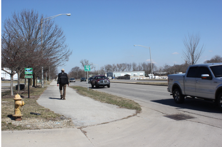
Existing Side Path along North 9th Street near Sagamore Parkway
