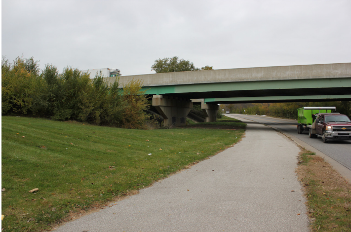
North 9th Street and Sagamore Parkway Overpass
