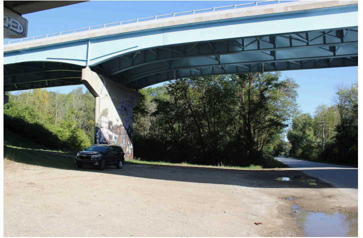
Location of Proposed Trailhead at North River Road under Sagamore Parkway Overpass
