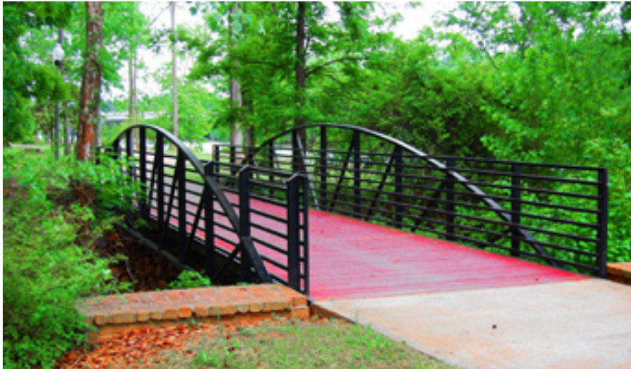
Concrete approach and bridge deck due to velocities
