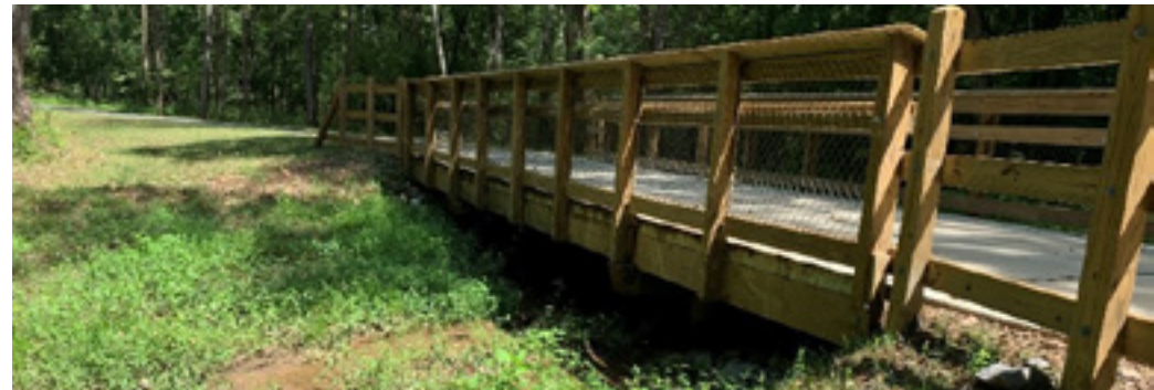
Example of small bridge constructed on-site for small drainage
