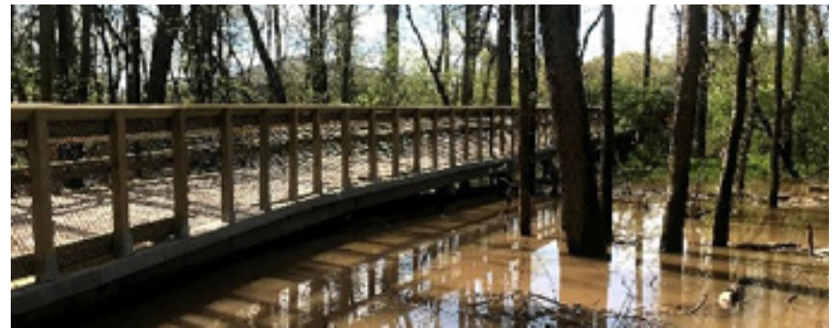
Example of top down constructed boulder through wetlands, a deck made of concrete for bikes, and 14-foot wide for maintenance vehicles
