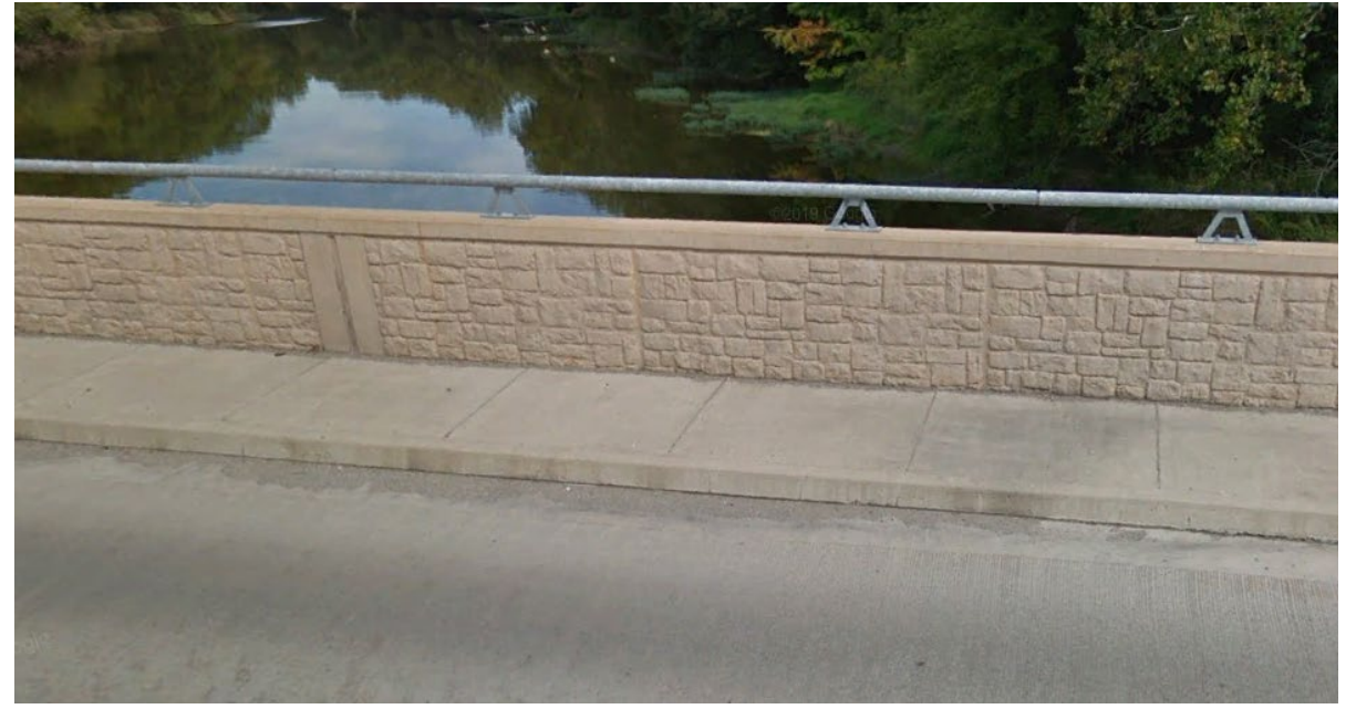
Concrete Bridge Railing Retrofit > 3.5 feet Height
